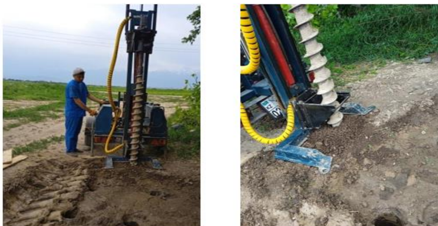
Fig. 1. Drilling of control wells after a single treatment.
